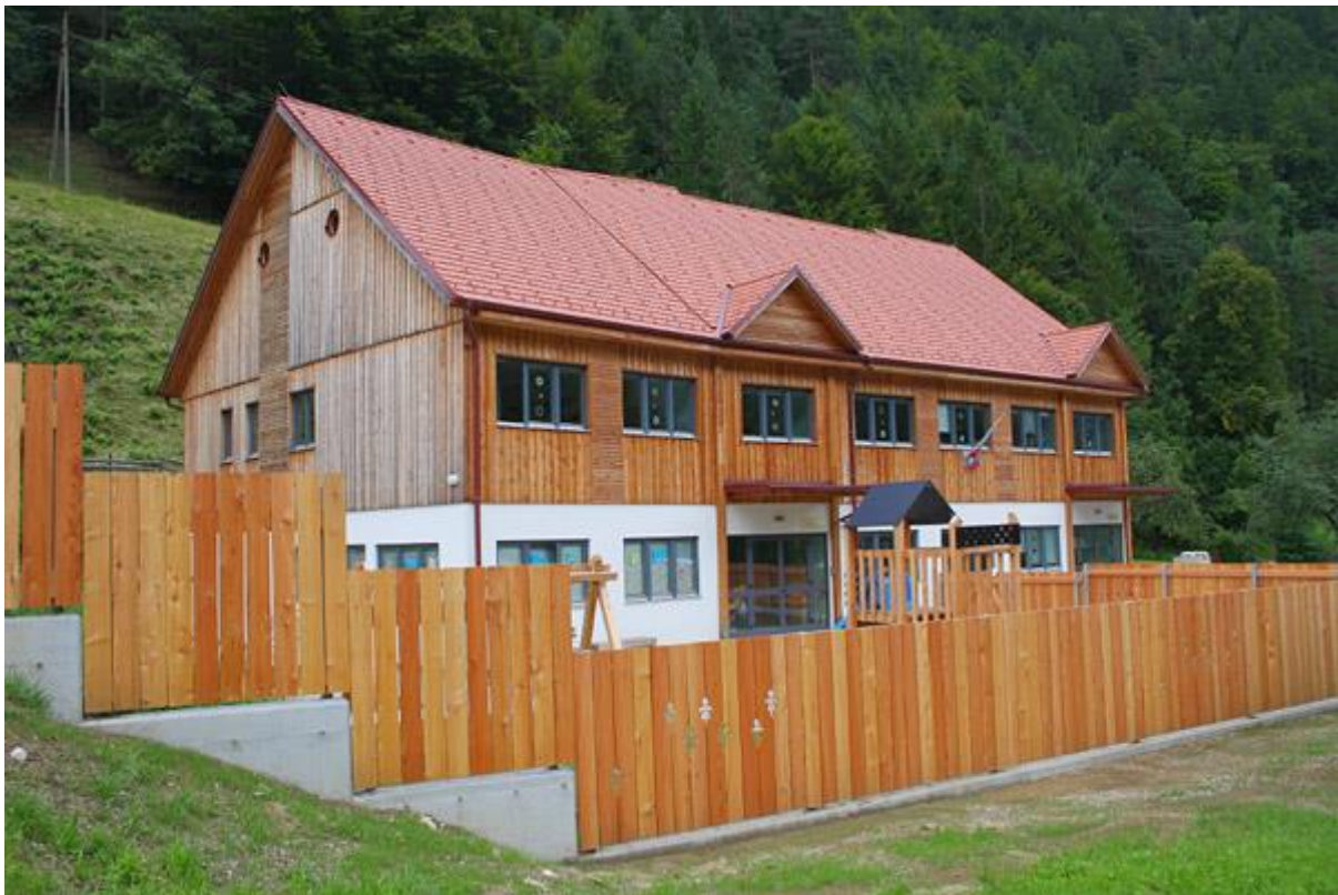
Figure 6: Mountain wood: Solčava primary school
