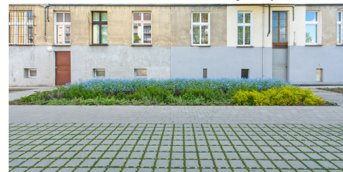
Demos construction, New green system, Wrocław
