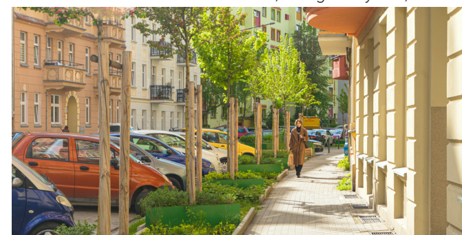
Demos construction, New green system, Wrocław
