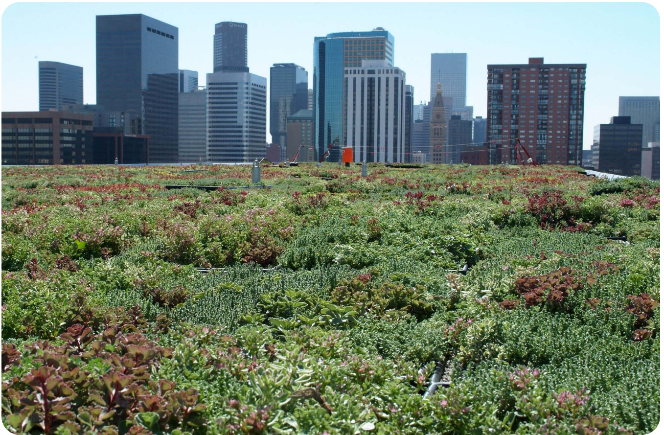
Photograph of a green roof in Denver, ©Wikipedia Commons CC BY-SA 3.0
