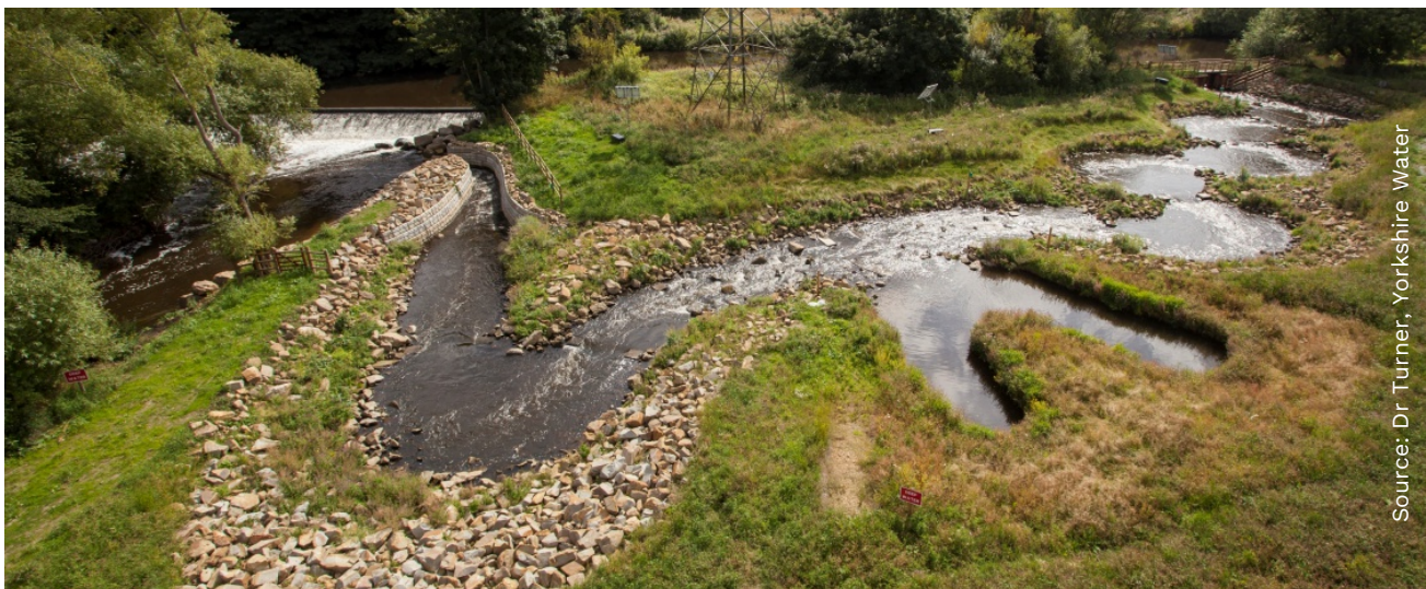
Figure 5: A natural bypass channel created alongside a strategically important barrier (Rodley Weir, UK)
