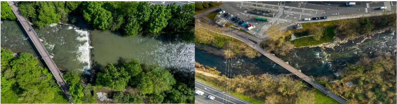
Figure 4: MERLIN Case Study 2 (Basque Country, Deba River) - removal of barriers with benefits for reducing flood risk (before and after implementation)
