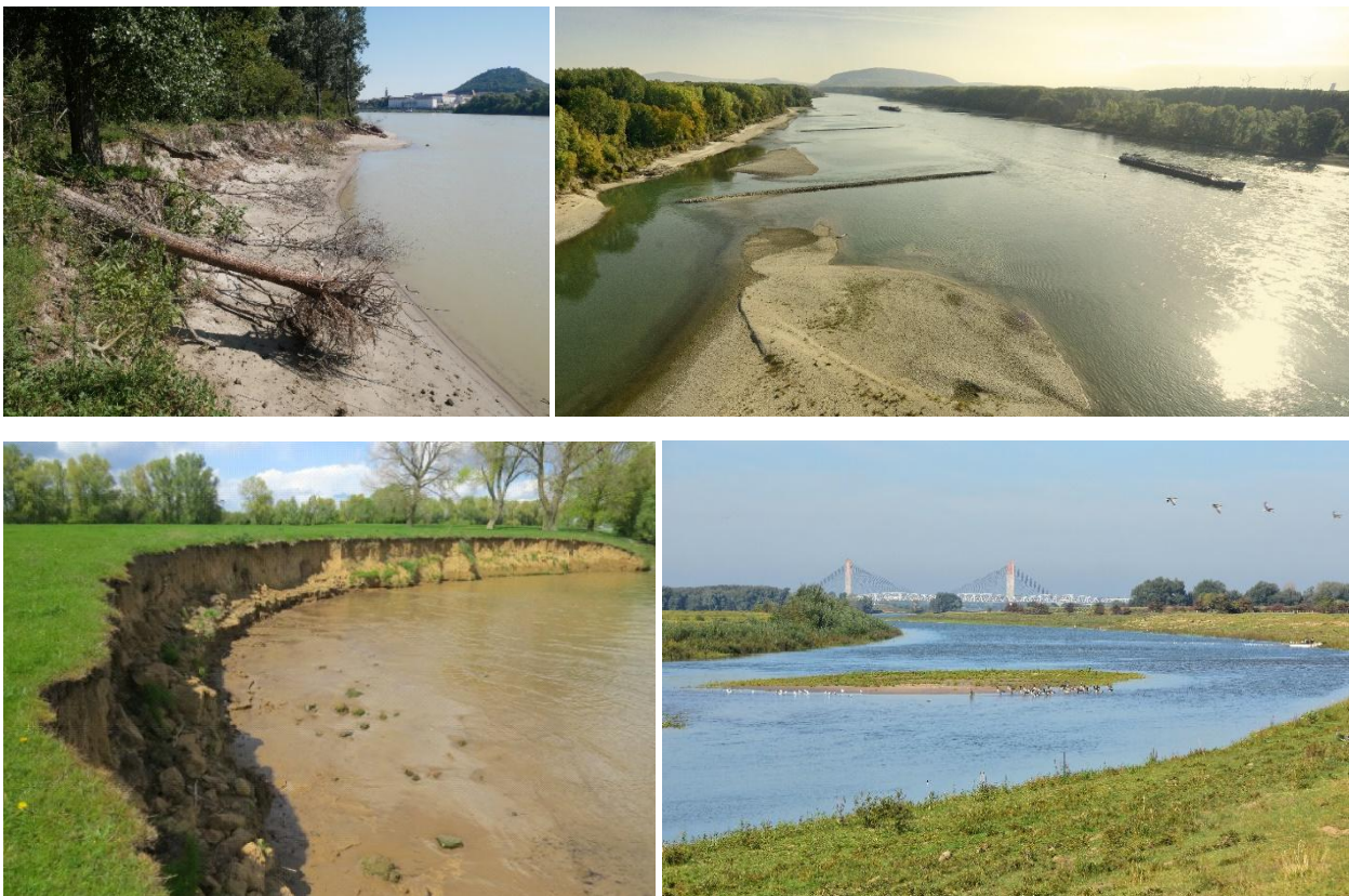
Figure 1 Examples of NbS for greening inland waterways. Top left bank protection removed (Danube, AT), top right adapted groynes (Danube, AT), bottom left bank removal protection (Meuse, NL), bottom right side channel reconnection (Rhine, NL)
