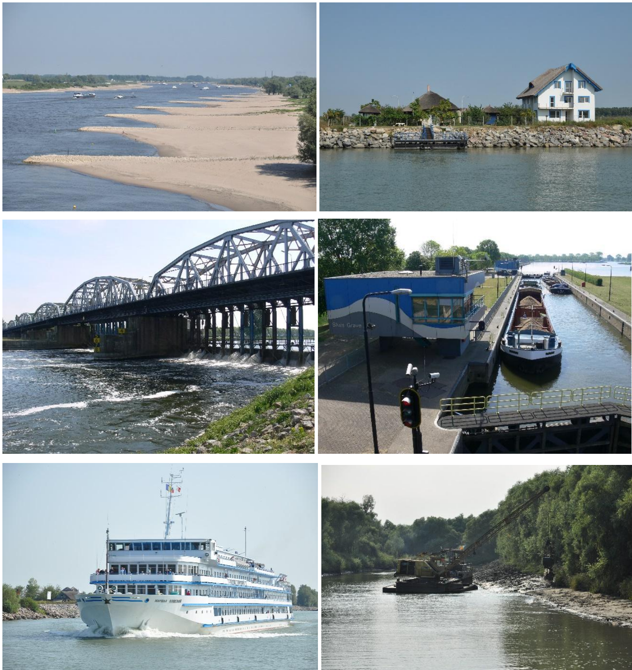
Figure 3 Environmental impacts of inland water transport. Top: standardising width and depth with groynes (left) and bank protection against erosion (right) modify habitats; Middle: weirs and sluices to regulate water depth disrupt connectivity and free-flow conditions; Bottom: waves and water displacement (left) and dredging (right) impact biota.
