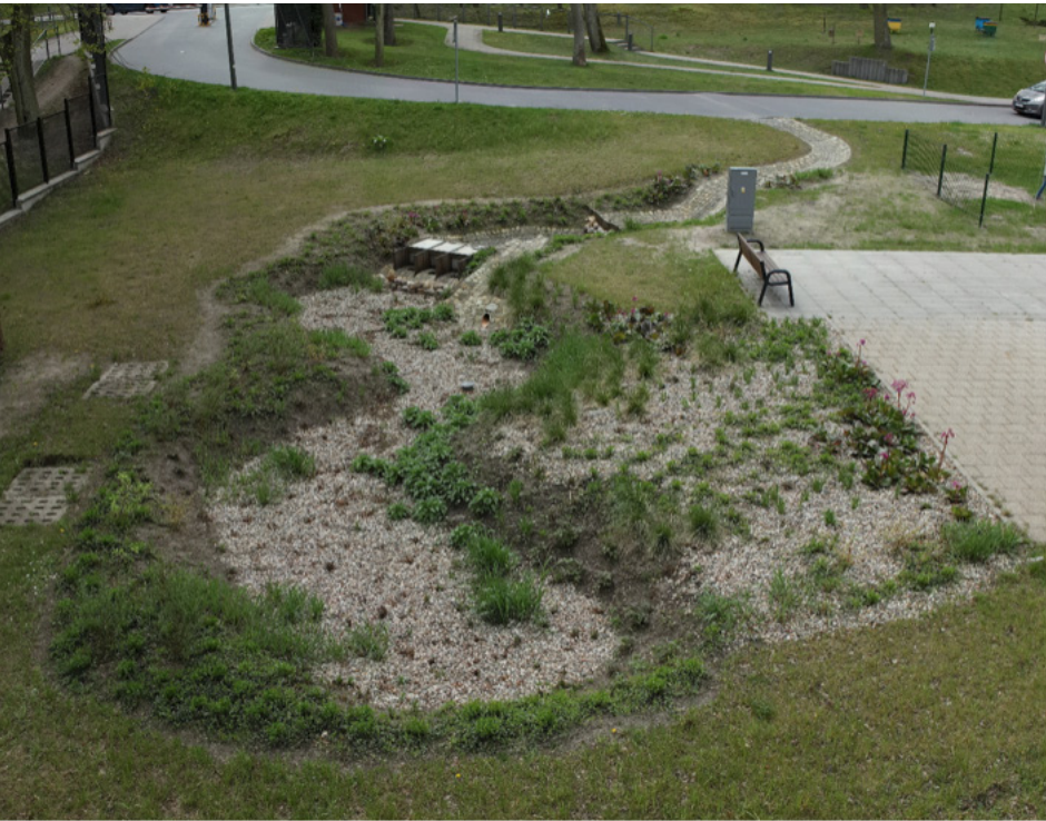
Figure 2.1.2 Design example of the rain garden system as implemented at the Urban Real Lab 9 site
