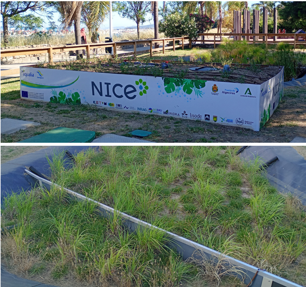
Figure 2.3.10 Installation photo of the storm water run off storage tank (top) and wetland basin for storm water treatment (bottom).
