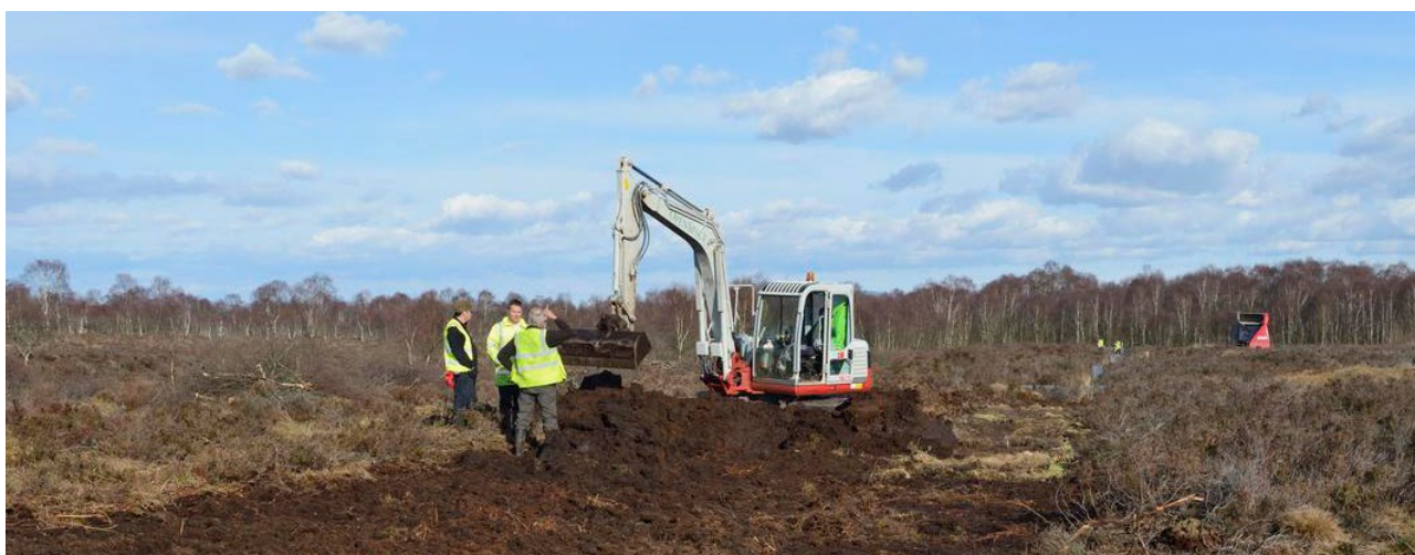
Demonstrating peatland restoration in action at Flanders Moss SAC site. © NatureScot
