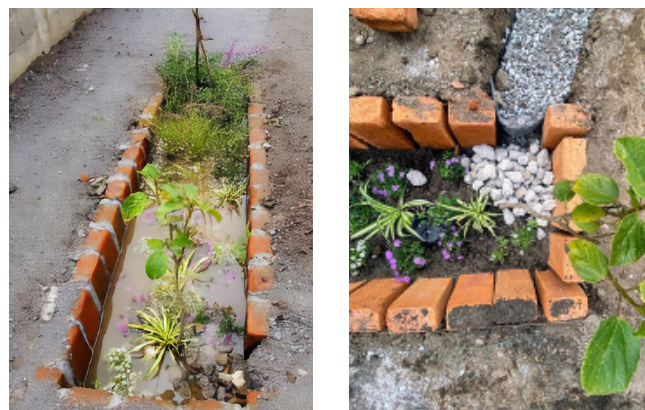
Niskotehnološka kišna bašta u Kitu (© YES Innovation)
